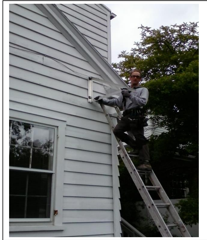
Mike making first aluminum angle brace attachments:
