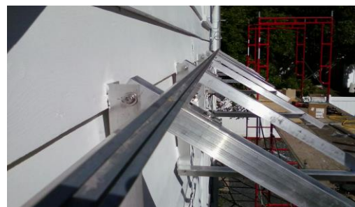
"Straight as a rail" - front-to-back tolerances for the frameless SunPrime mounting was only 1/4"
